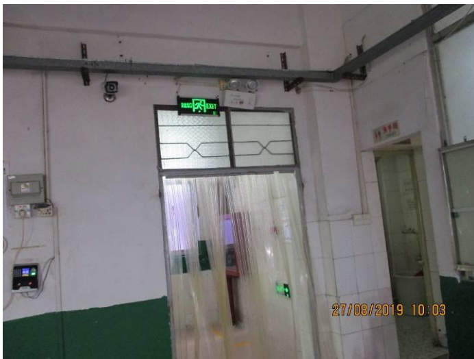
Emergency exit marked with emergency light and exit sign
